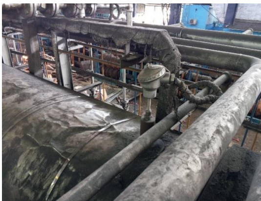
Gambar 4. Sensor Termokopel Zone 2B
