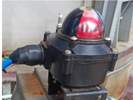
Gambar 2.14 Function Box Solenoid Valve
