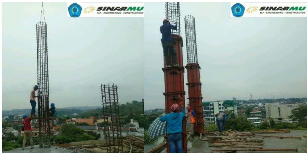
Fig. 7. Installation of steel bar and formwork
