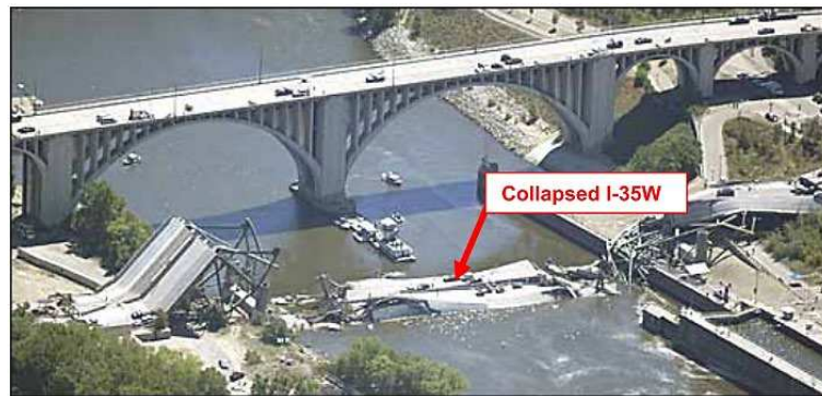
Figure 2. Photograph of the I-35W Bridge Collapse [2]
