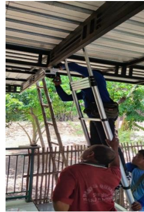
Gambar 3.3 Pemasangan Hardware Smart Lighting
