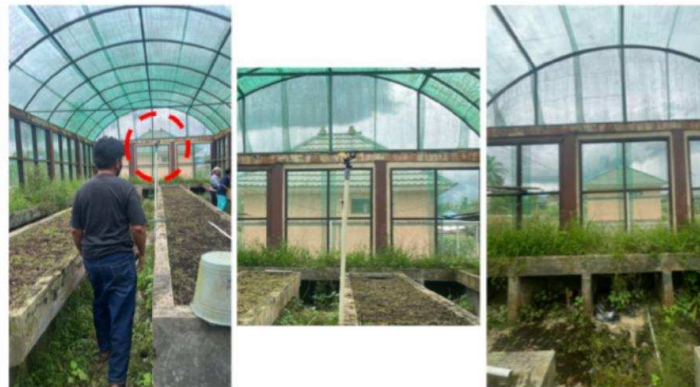
Figure 2. Initial condition of the TTP greenhouse showing the sprinkler system causing uneven water distribution and inefficient irrigation.
