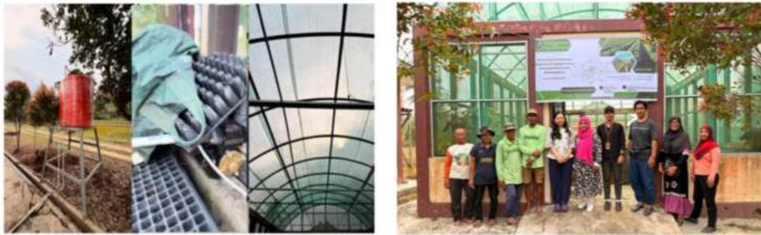
Figure 5 Installation of key greenhouse infrastructure and community training session with local farmers at TTP
