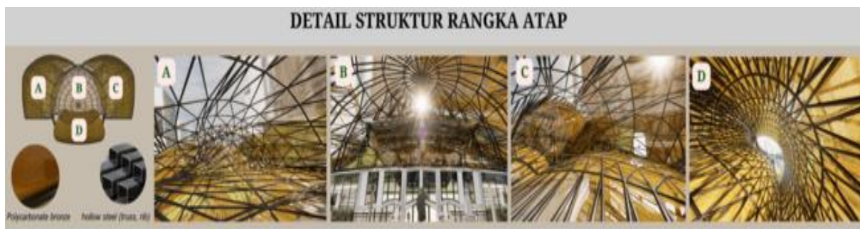
Gambar 7. Detail Struktur Rangka Atap Garuda Tourist Information Center
