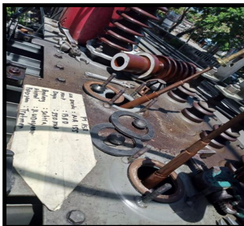
Gambar 12. Penggantian Seal/Packing Trafo
