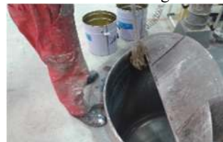
4. Re-scrap the tank using a long brush.
