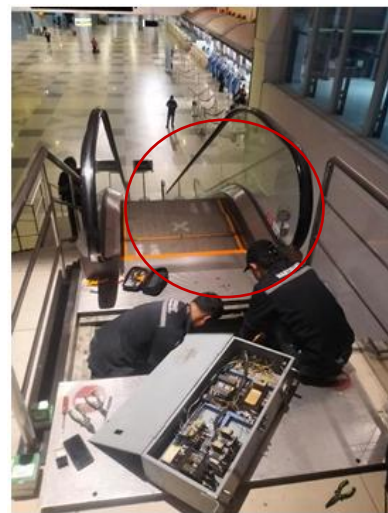
Figure 5. Escalator Observation (Source: Author documentation, 2024)
