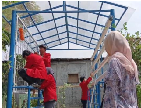
Figure 1. Hydroponic Installation Activities
