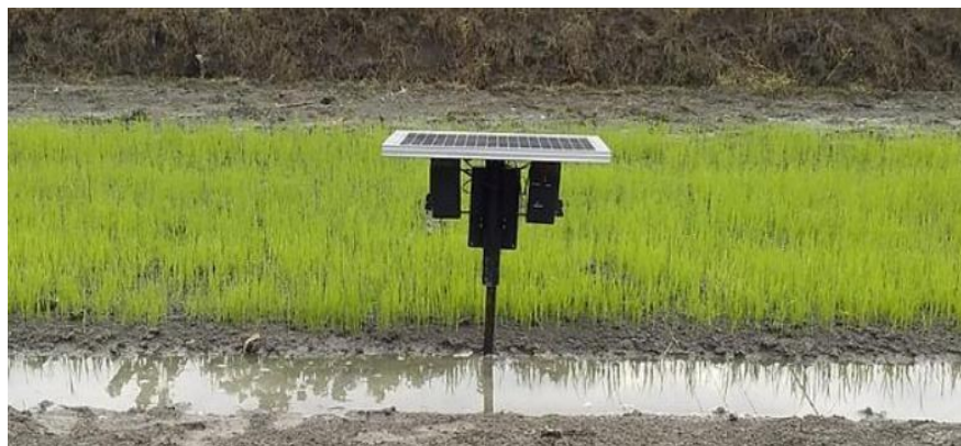
Figure 5. Installation of the solar-powered ultrasonic pest repellent in the rice field
