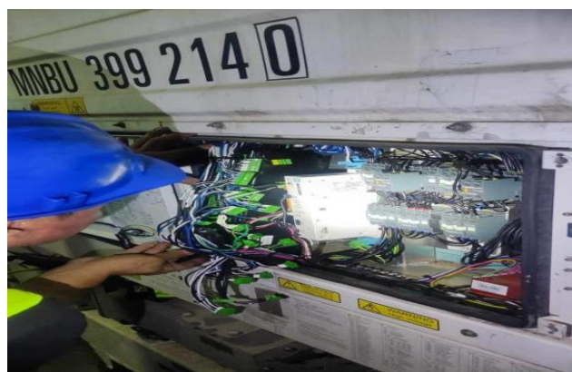
Figure 3. Repair on control box by reefer technician
