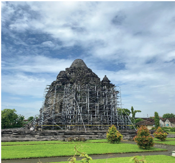
Figure 1. Restoration of Kalasan Temple in progress
