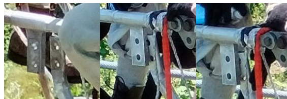
Figure 11. Cleaning Dirt from the Jumper Clamp
