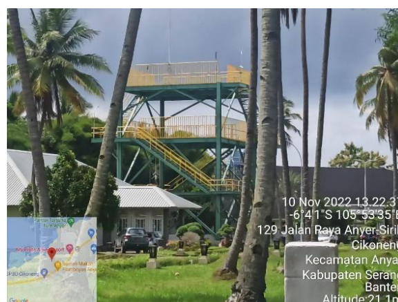
Figure 5. One of the shelters on Anyar Subdistrict (Source: Research Result, 2022)
