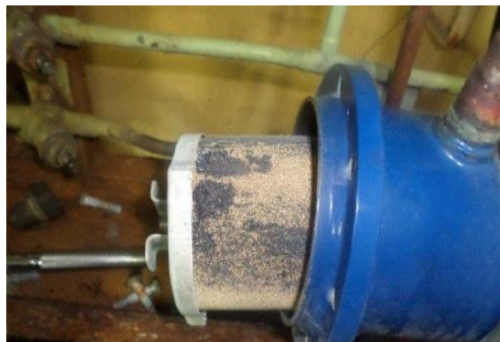
Figure 1. Filter dryer kotor
