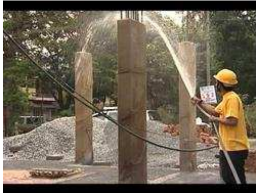
Gambar 8. Proses Curing
