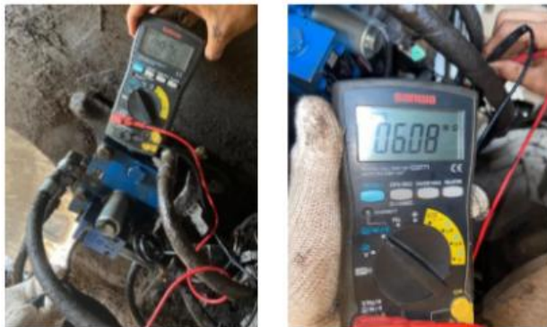
Figure 4. EPC Hoist HEPC Solenoid Measurement
