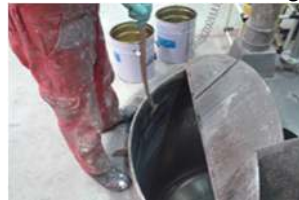
3. Scrap the tank using scrapper.
