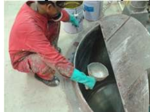
5. Flush the tank using dirty thinner.
