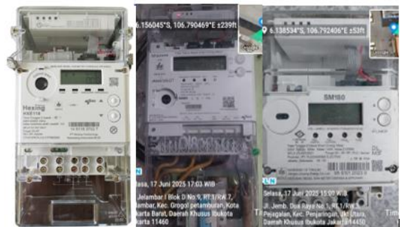
Figure 3. AMI enabled kWh meter
