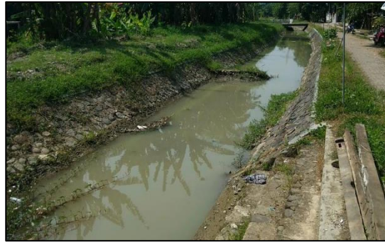
Fig. 3. Existing Condition Hm 50+00
