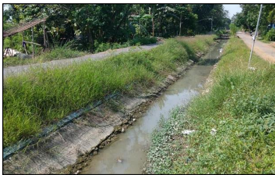
Fig. 4. Existing Condition Hm 58+00
