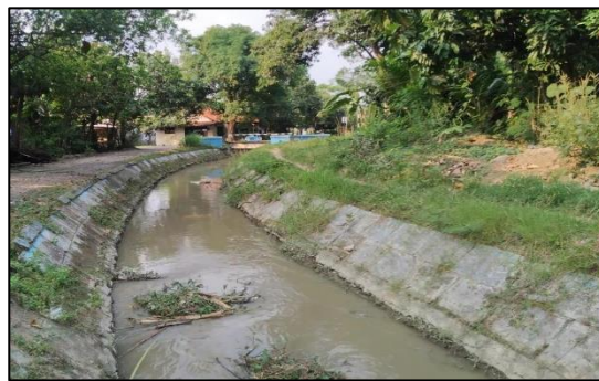
Fig. 5. Existing Condition Hm 71+00
