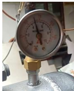
Figure 2. Observation of the pressure outlet from the ammonia condenser.
