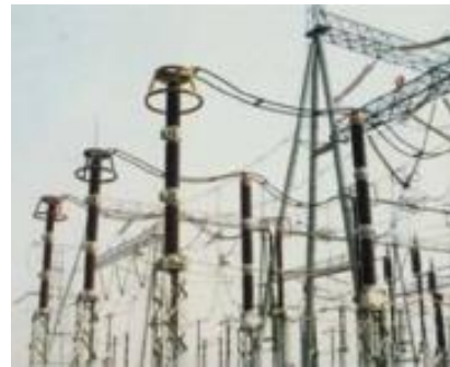
(Gambar 2.1 Lightning Arrester )
