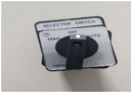
Gambar 6. Main Auto Selector Switch
