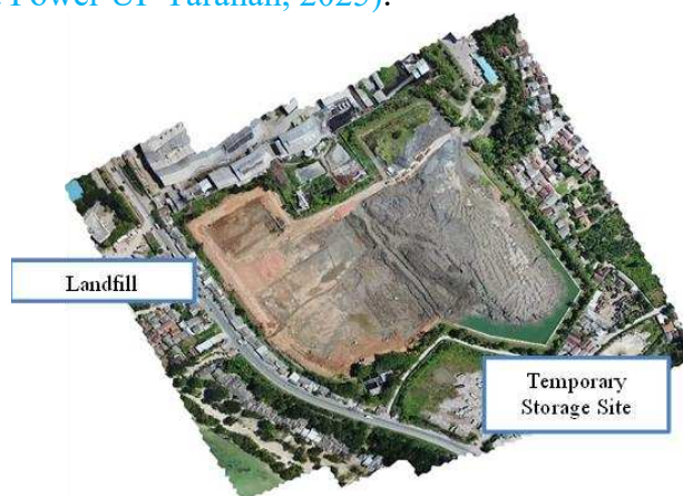
Figure 3. Layout of FABA Management Facility of PLTU Tarahan.
