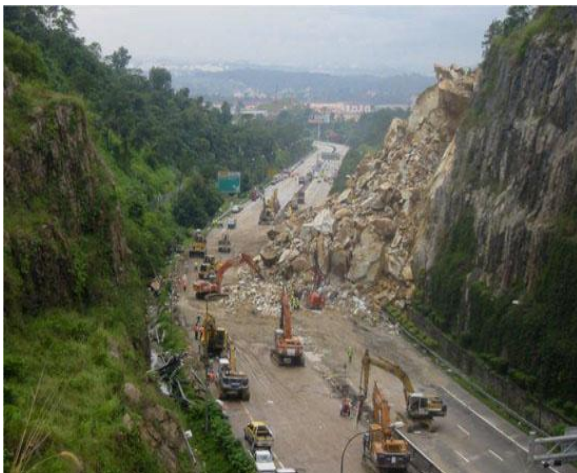
Figure 2. The rock slope failure incident at the Bukit Lanjan Interchange (KM 21.8 of NKVE) on November 26, 2003. The entire expressway was closed to the public due to the failure of materials obstructing the road [33].
