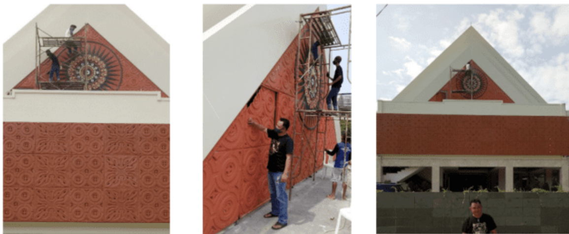
Figure 17. Application of Toraja Motifs on Relief Design of Aesthetic Elements for Building Façade [by Gustyan Rachmadi, 2020, Steel Construction Resin]
