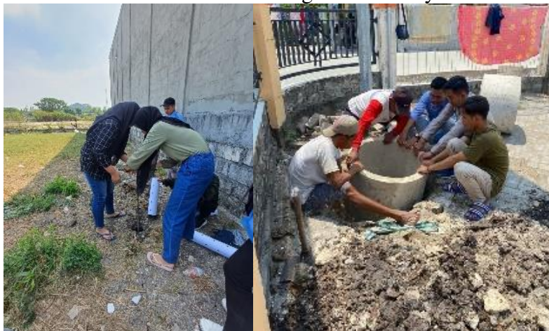
Figure 4. Installation of Biopores and Infiltration Wells in collaboration with the Blawi Village Community.
