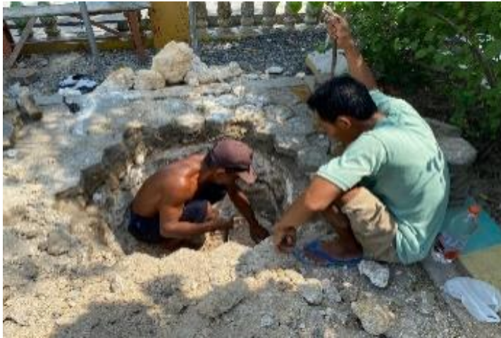
Figure 3. Infiltration Well Digging Process.
