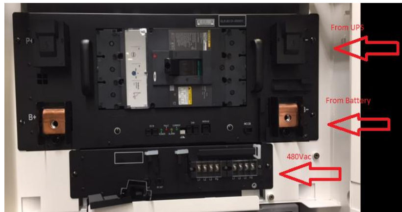
Figure 2. BCU with Optional Auxiliary Breaker Switch
