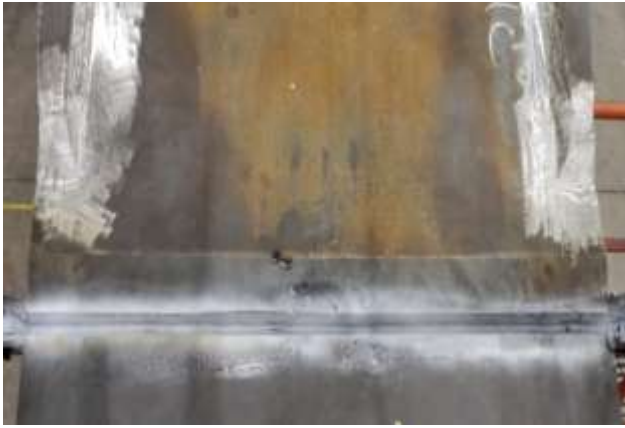
Fig. 6. Welding Seam After MPI Checking
