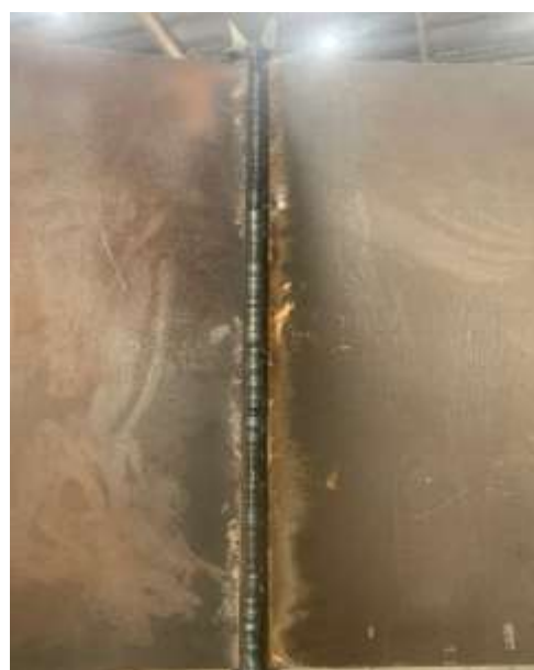
Fig. 5. Welding Seam After Back Gouging Process
