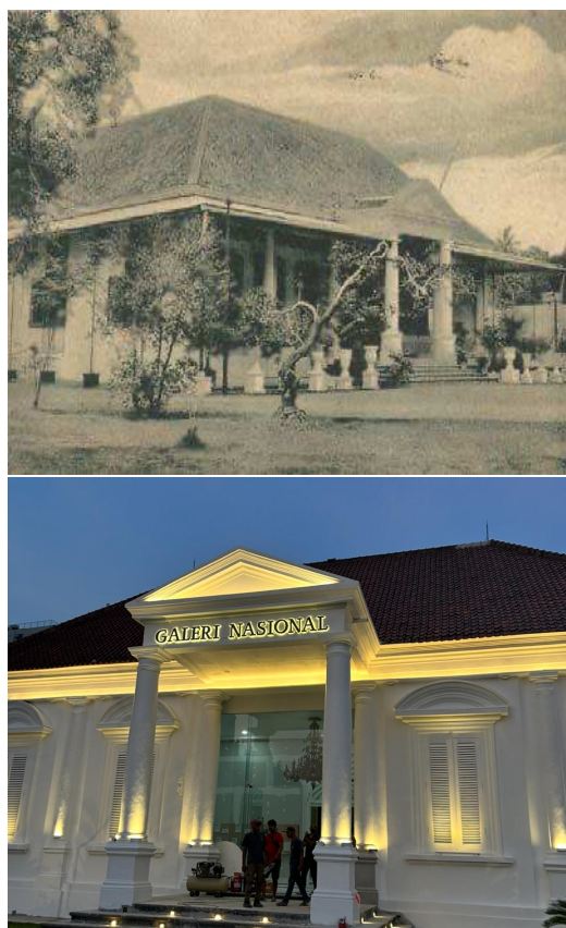
Figure 10. GNI Building as a Female Dormitory in 1905 and GNI Today [Source: GNI Documentation]
