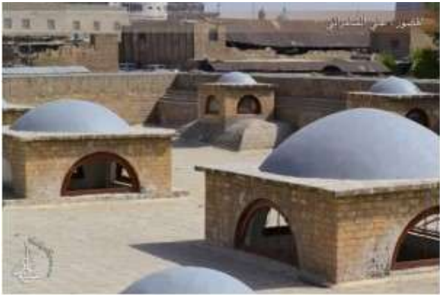
Figure 9. The skylight in the Mustansiriya Madrasa [23]
