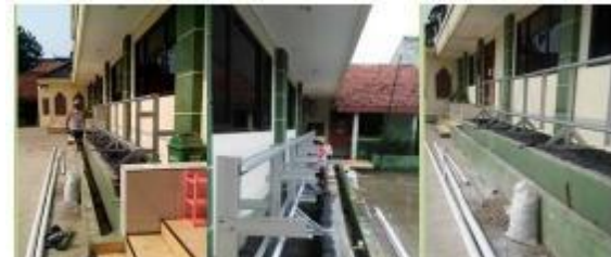
Fig. 8. Stage 3: Making Construction with Canal C Steel and Finishing of Fish Pond (Source: Team's Documentation, 2017)
