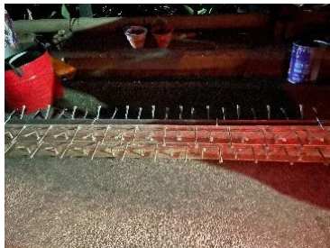
Gambar 2. Sambungan Tipe Strip Seal
