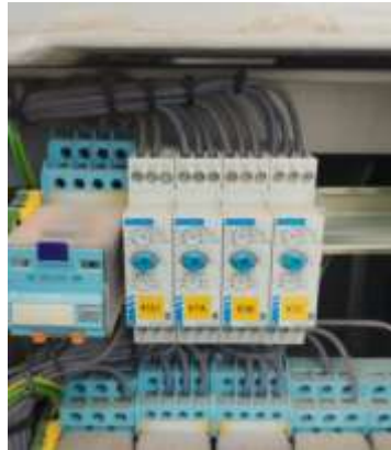
Figure 8. KT 6.1 Timer (Pole Discrepancy)
