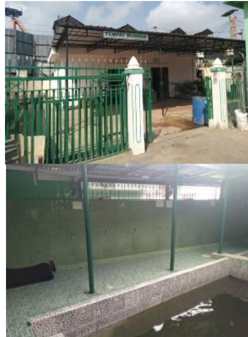
Figure 13. Ablution Facility (Source: Author's Document, 2025)
