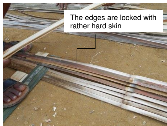
Figure 5. The process of weaving bamboo walls.
