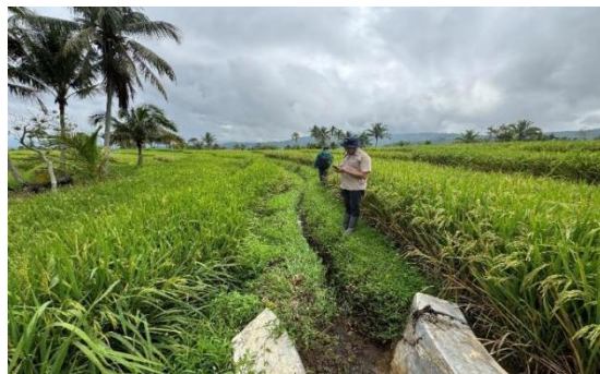
Fig. 5. Condition of Primary and Secondary Canals in the Bdr. Ambacang Irrigation Area
