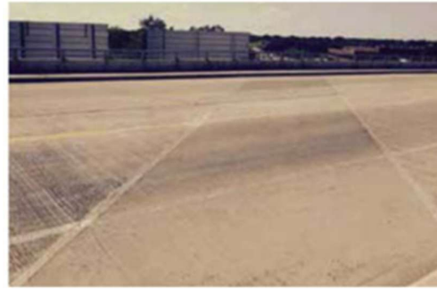
Figure 7 Successful study of the application of ECC on Linkslab using ECC on the Grove Street Bridge (Boughanem et al., 2013; Yildirim, 2018; Yin et al., 2019).
