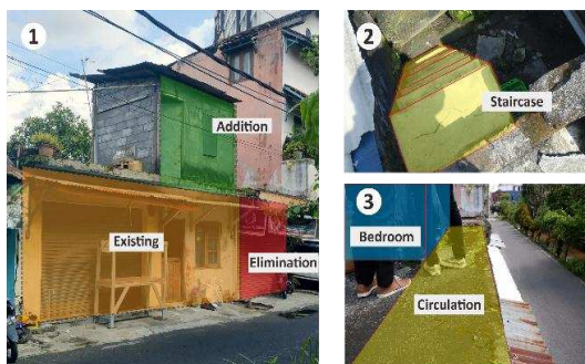
Figure 5. (1) Limited vertical addition & partial elimination of existing mass in case 5; (2) Non-standard staircase with steep inclination due to spatial constraints; (3) Narrow circulation leading to the bedroom, lacking safety barriers despite level differences
