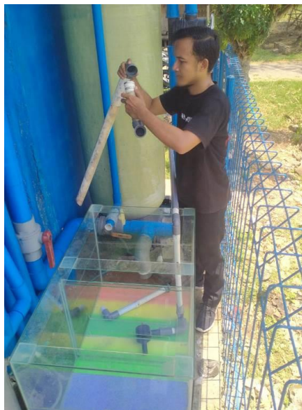
Gambar 2. Proses pemasangan filter MBG
