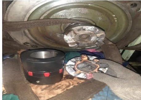
Figure 6. Damage to the rubber coupling Source: Researcher's documentation (2023)
