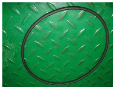
Figure 7. Damage to the oil seal Researcher's documentation (2023)
