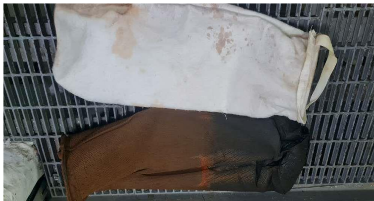
Figure 7. Replacement of OWS filter bag Source: Research Document
