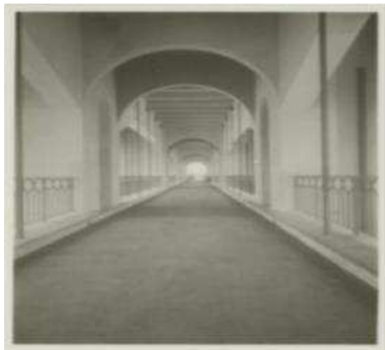
Figure 1. Walahar Dam, Karawang, interior view
