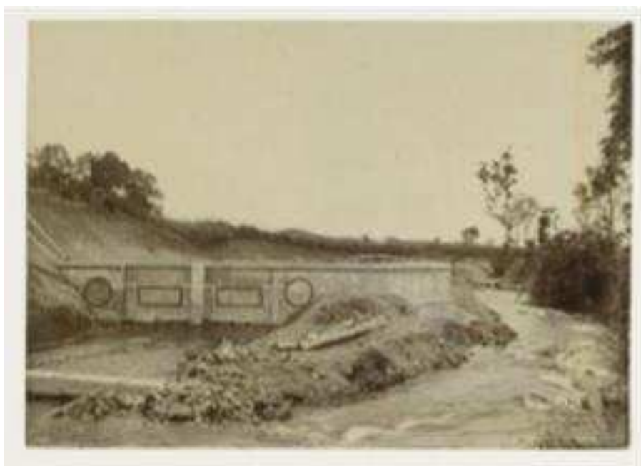
Figure 4. Pematangsiantar Dam (East Sumatra), 1921
